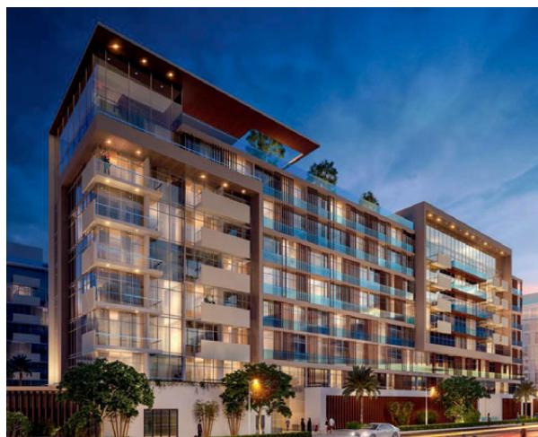
Construction activities on Phase 4 of Azizi Riviera will begin in July 2018.
